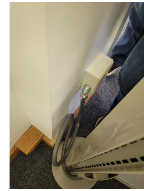
TYPICAL EXISTING POWERED FURNITURE SYSTEM POWER CONNECTIONS SHOWN. TO BE DISCONNECTED AS NOTED FOR RELOCATION.
