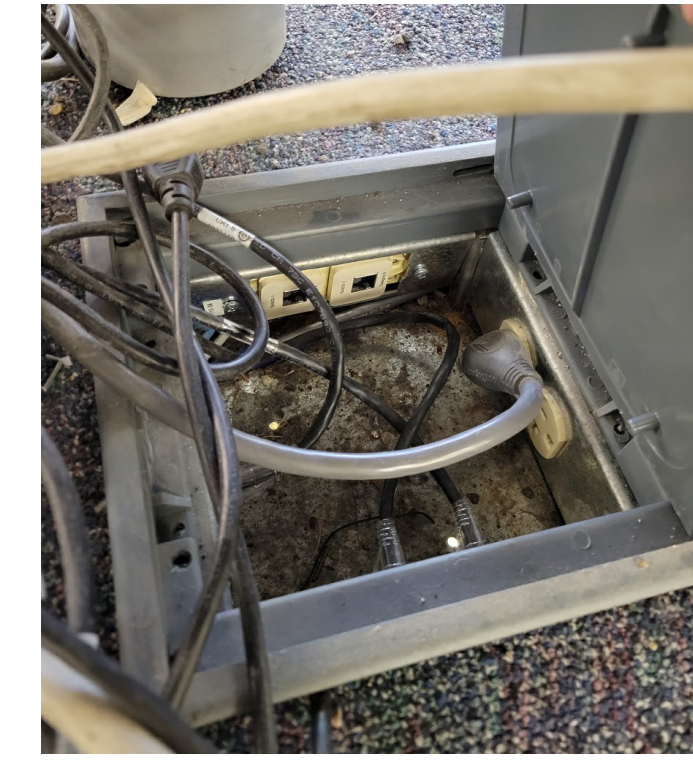
TYPICAL EXISTING FLOOR BOXES, TO BE MODIFIED WHERE NOTED FOR HARDWIRED FURNITURE WHIP CONNECTION.
