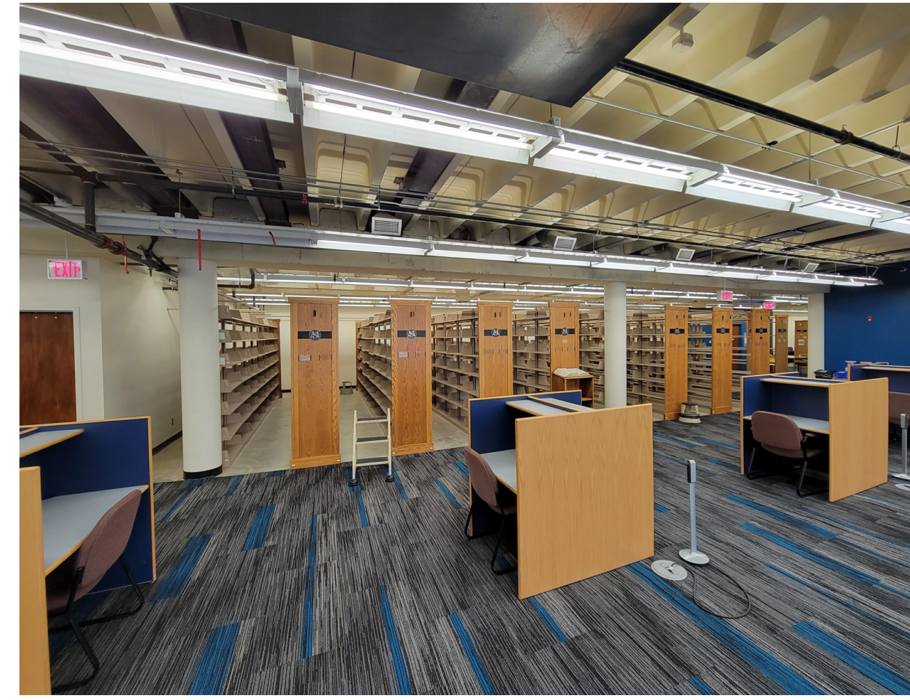
LEVEL 4 SPACE PICTURED. EXISTING STACKS TO BE REMOVED. NEW CARPET, FURNITURE, AND UNDERCARPET POWERED TRACK SYSTEM WITH FLOOR BOXES TO BE PROVIDED BY OTHERS. ELECTRICAL CONTRACTOR SHALL BRING 120V POWER CIRCUIT TO UNDERCARPET SYSTEM.
