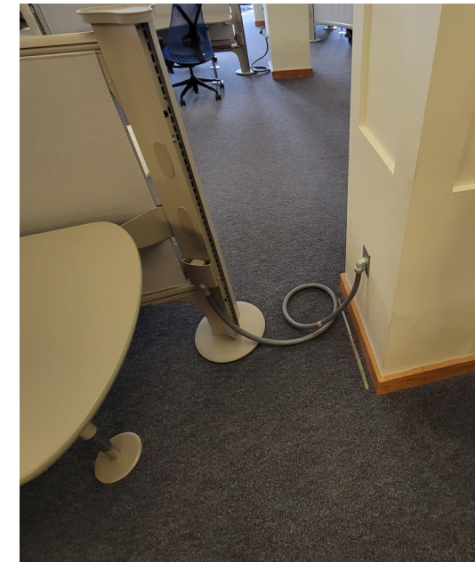
TYPICAL EXISTING POWERED FURNITURE SYSTEM POWER CONNECTIONS SHOWN. TO BE DISCONNECTED AS NOTED FOR RELOCATION.
