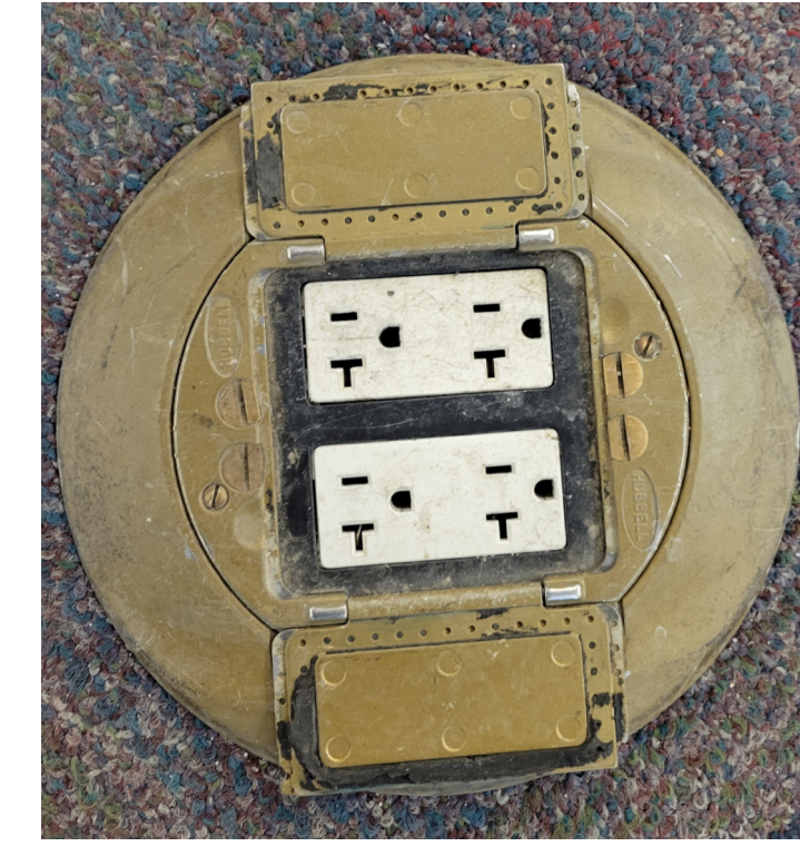
TYPICAL EXISTING FLOOR BOXES, TO BE MODIFIED WHERE NOTED FOR HARDWIRED FURNITURE WHIP CONNECTION.
