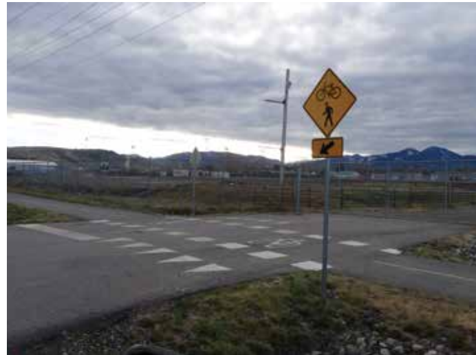
Pavement markings and signage on Oak Street (WTI)
