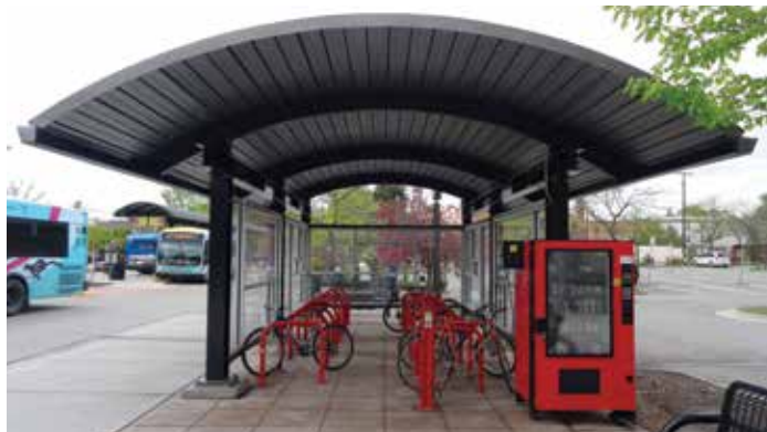
Covered bike parking combined with a vending machine
