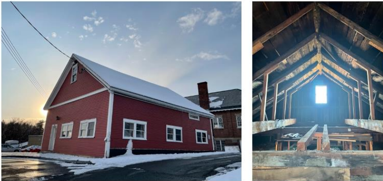
Figure 1. Images of the exterior (left) and interior (right) of Kimball Barn as it stood on the KUA campus in December 2021 shortly before deconstruction began.
