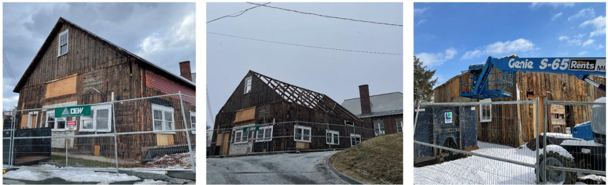
Figure 2. Images of the Kimball Barn during the deconstruction process.
