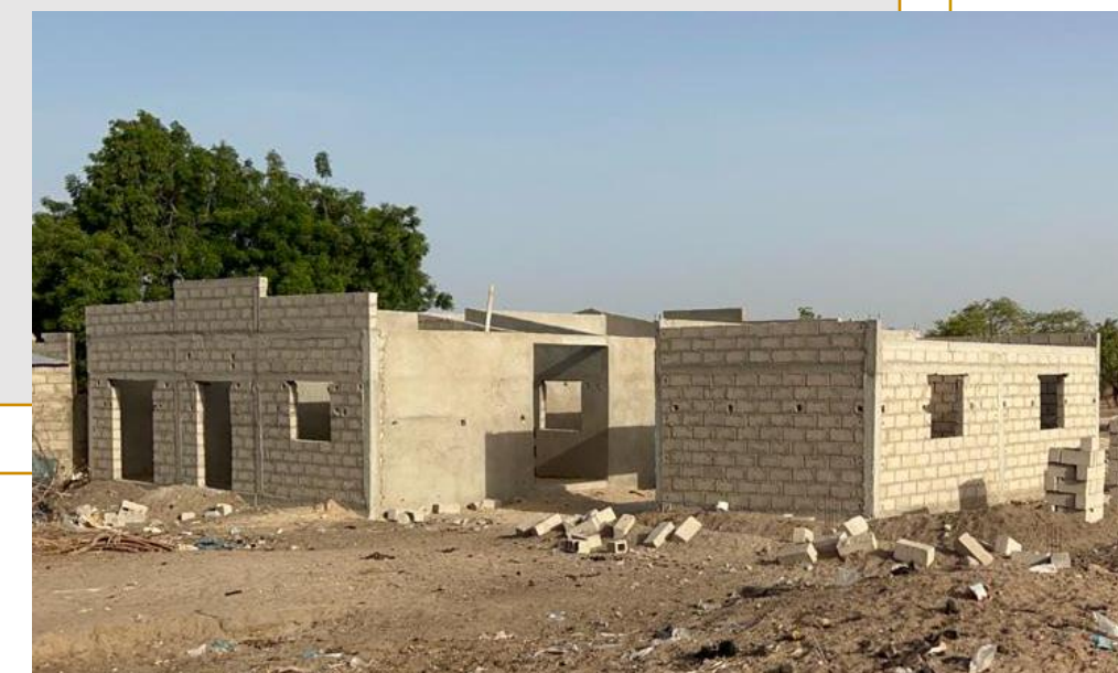
Figure 1: Construction of food processing plant in Ndangane
