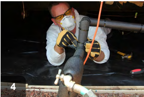
4 Fasten insulation to water lines with zip ties
