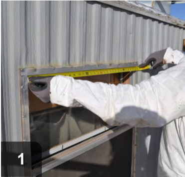
1 Measure sash for width of replacement glass -- cut glass to 1/4" less than sash width
