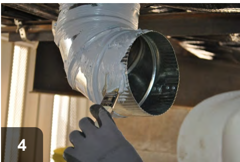
4 Apply mastic to all elbow joints and flange
