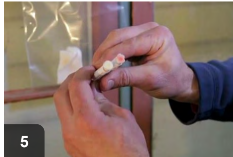
5 Red indicates lead positive. White indicates lead negative
