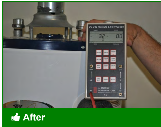
Test to verify combustion appliances are within depressurization limits
