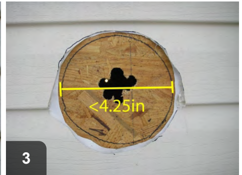
Clear wall surface and mark hole size 1/4" larger than termination fitting
