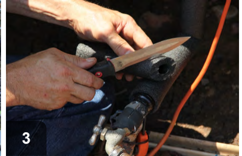
3 Measure and cut insulation to fit water lines. Miter insulation at elbows and tees
