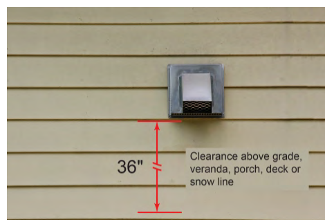
Install vent at least 36" above grade, porch, deck, veranda, or snow line
