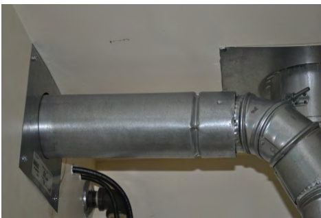
Inspect ventilation systems for inadequate slope
