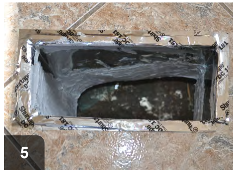
After securely fastened, duct should be sealed with mesh and mastic
