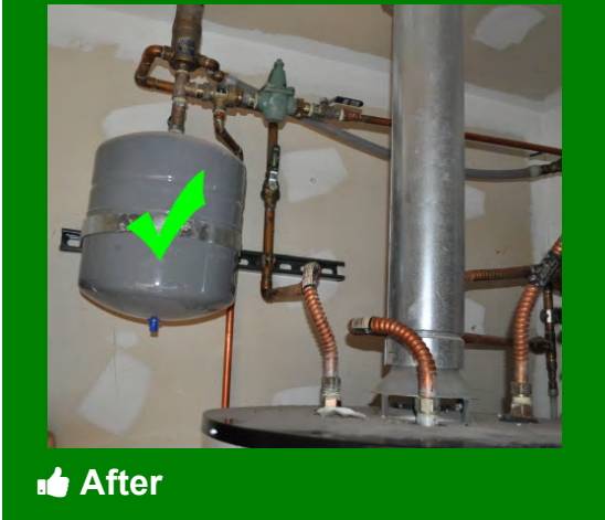
Potable water expansion tank
