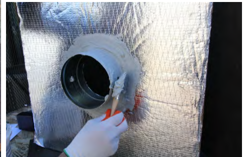
Apply mastic liberally and install flex duct
