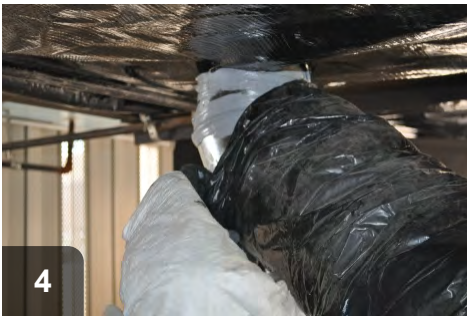
4 Slide insulation and outer casing over metal ducting
