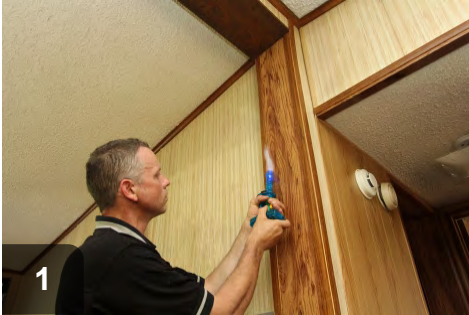
Identify leaks in marriage line using a blower door and smoke
