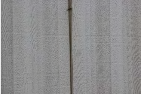
Seams on aluminum siding must be tight.
