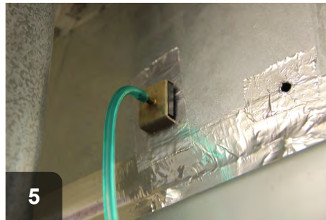
Probe placed after the coil.
