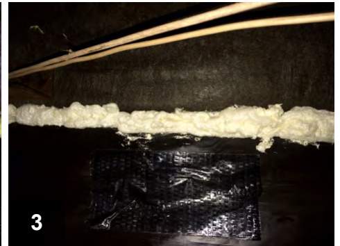
3 Apply foam or caulking over backer
