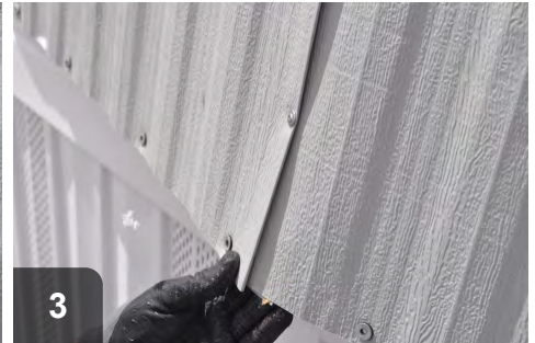
Seam should remain together with temporary fastener
