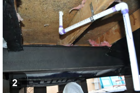
2 Cavities should be completely cleared of debris
