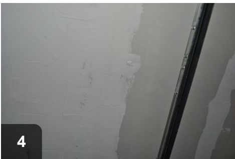
4 Add joint tape and coat of joint compound
