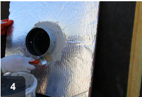
4 Coat joint between starting collar and duct board with mastic. Liberally coat the metal collar where flex attaches
