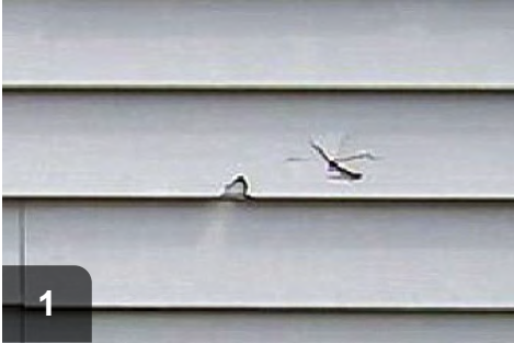
Replace damaged siding
