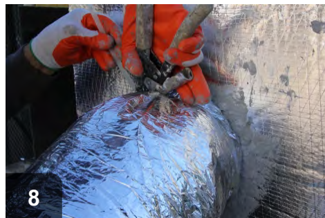
8 Pull insulation over duct liner and secure with a zip tie.
