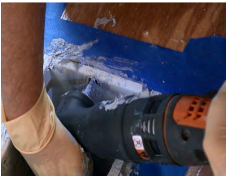
Mechanically fasten the boot to the subfloor.
