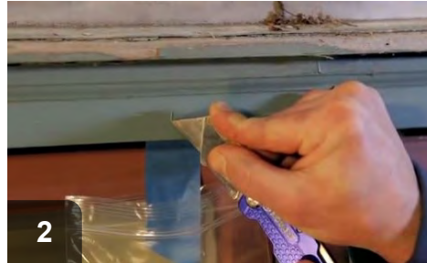
2 Cut sample site at an angle to expose all older paint layers
