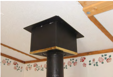
Proper clearance to combustibles will be maintained through the roof assembly.
