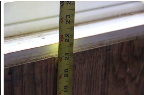
Window sill height is within code guidelines.
