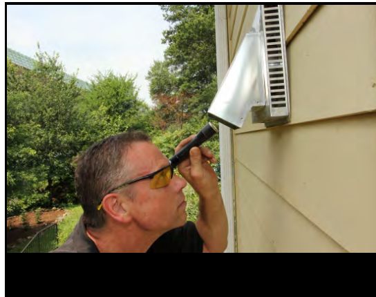
Inspect direct venting for proper connections, rust, corrosion, and clearances
