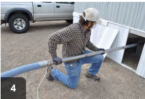
Proceed with blowing insulation without fear of static shock
