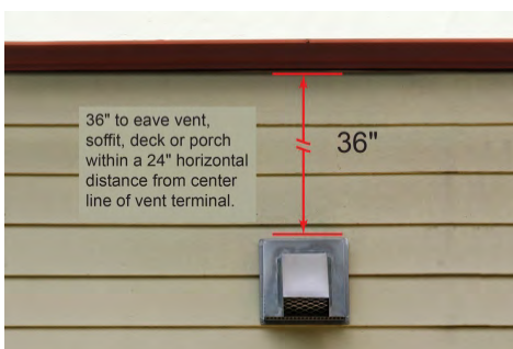
Install vent terminals at least 36" below any eave, soffit, porch, or deck within 24 horizontal inches of center of vent
