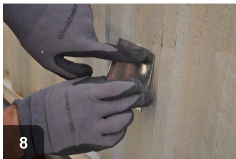
Flex patch to contour to wall
