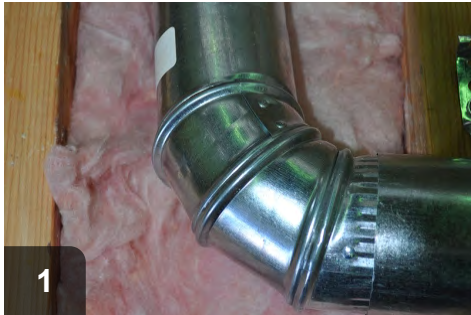
1 Prepare work area by assessing any safety concerns
