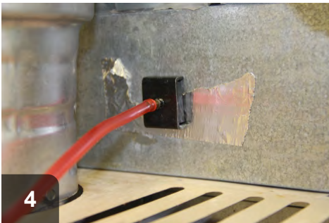
Probe placed before the coil.
