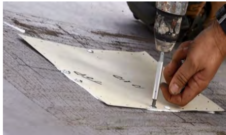
Secure the metal patch to the roof being sure to place mechanical fasteners through the sealant.
