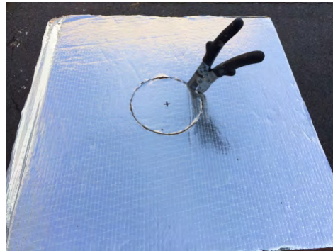
Cut the proper size hole in duct board
