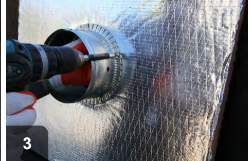
3 Fasten the collar to the backer ring by driving at least three equally spaced screws through the collar, duct board
