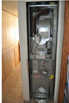
Test undiluted flue gases in induced-draft furnaces
