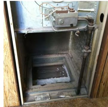
Inspect plenum for damage, then clean, scrape, and seal
