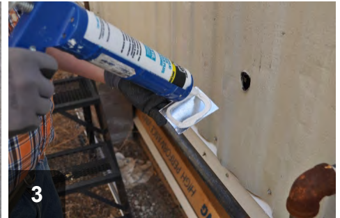
3 Apply sealant to back of patch to maintain air barrier
