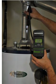
Complete carbon monoxide testing using a CO detector
