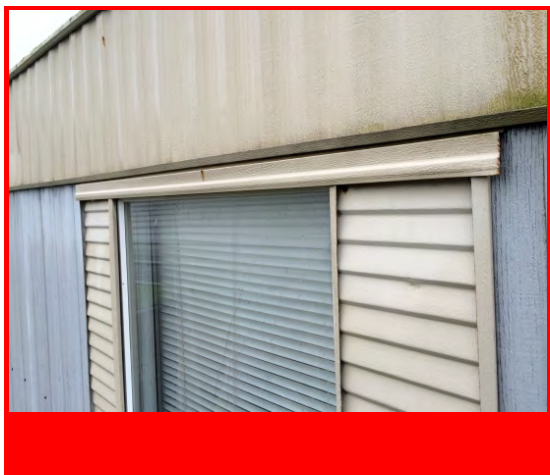
Install and caulk drip caps over manufactured home windows
