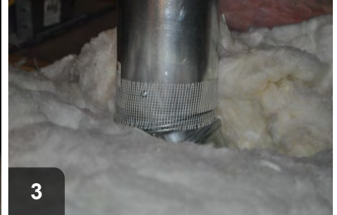
3 Then joints should be secured with fiberglass tape
