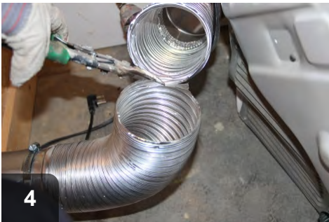
4 Trim metal vent to ensure the run is as short and straight as possible.
