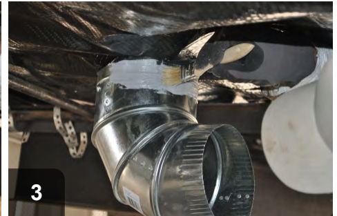
3 Apply mastic at metal-to-metal connection
