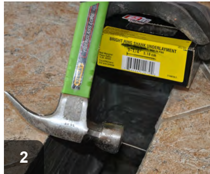
Use ring-shank nails to hold ducting in place to subfloor
