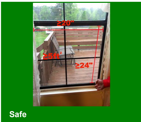
Egress window in bedroom of manufactured house
