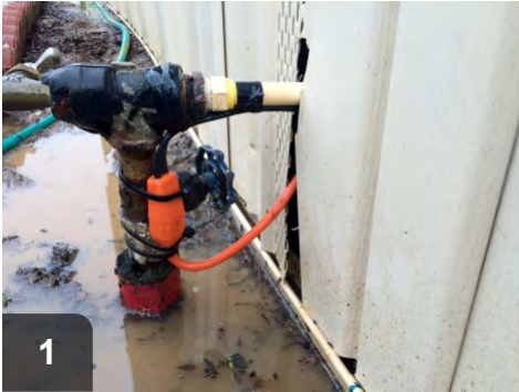
1 Install thermostat in firm contact with the pipe at the coldest point
