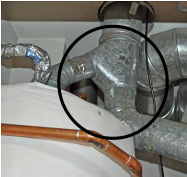
Common vent of natural draft appliances highlighted
