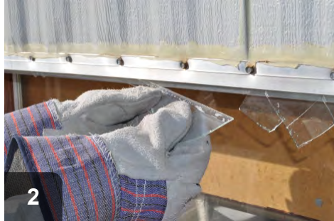
2 Wearing protective gloves, remove large glass pieces carefully
