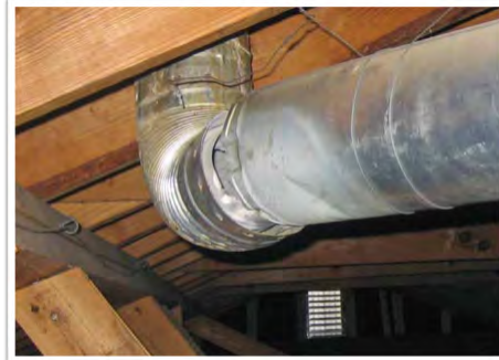
Inspect ventilation systems for damage
