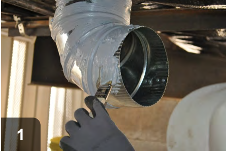
1 Apply mastic to flange
