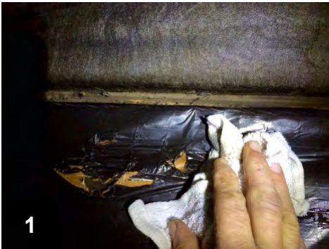
1 Clean belly wrap before air sealing
