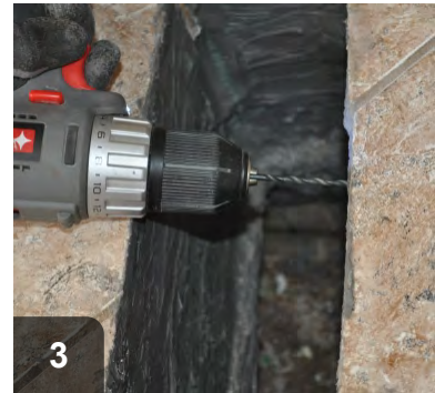
Drill pilot holes for metal fasteners
