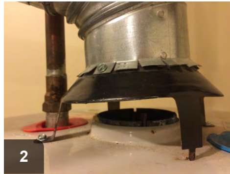
2 Check draft diverter alignment
