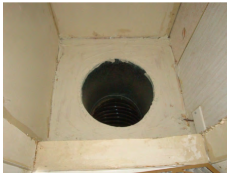
Apply mastic to inside seams of plenum
