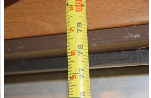
Egress doors are the proper height for egress.
