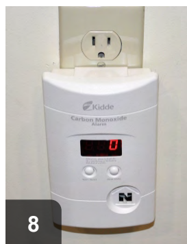
8 Verify safe levels on more than one instrument and in more than one location
