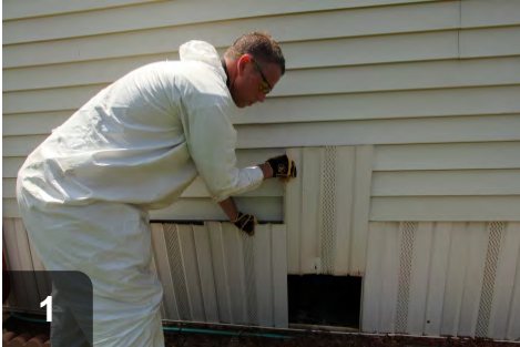
1 Remove skirting as needed for access to crawlspace
