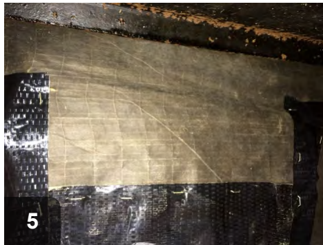
Apply belly repair tape and fasten with outward clinching (stitch) staples. Spray adhesive will help adhere the tape
