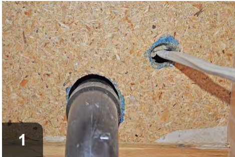
Prepare work space by removing any insulation
