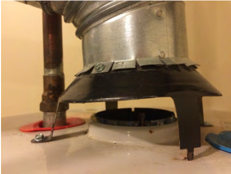
Check draft diverter alignment
