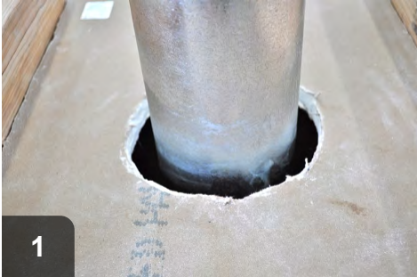
1 Prepare work area by removing any insulation and debris
