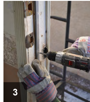
3 Install new weatherstrip
