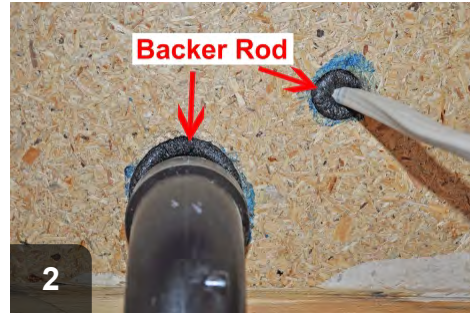
Infill with backer rod
