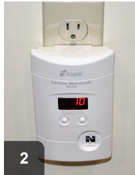
2 All homes should have CO monitors installed. If levels are elevated, look for the source
