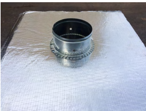
Insert the starting collar, bend tabs over and install at least 3 screws through the collar, duct board, and backer ring
