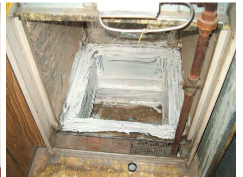
Plenum to duct trunk connection coated with mastic sealant
