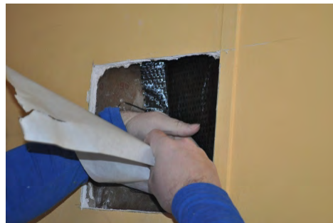
Repair vapor barrier
