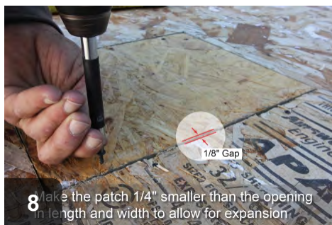
Fasten with 2" deck screws
