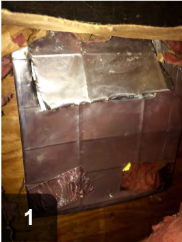
Thoroughly clean duct with solvent before applying foil tape and mastic
