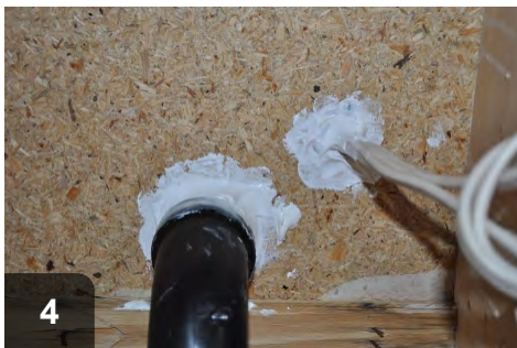
Visually inspect to verify no gaps remain
