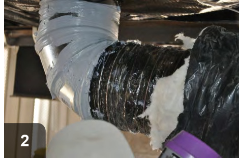
2 Slide inner liner onto flange with sealant
