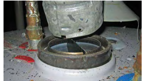
Inspect ventilation systems for disconnected pipes
