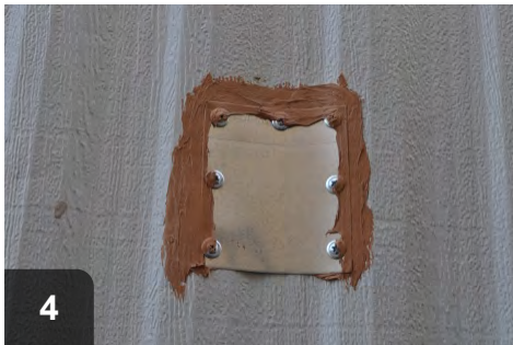
4 Ensure that patch is securely fastened and water-tight
