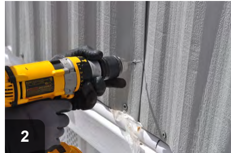
Temporarily fasten siding panels at joint to hold seam together
