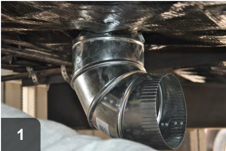
1 Attach elbow duct and orient in correct direction to minimize duct run
