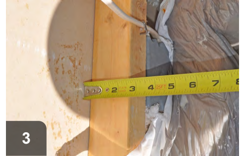
3 Measure depth of cavity
