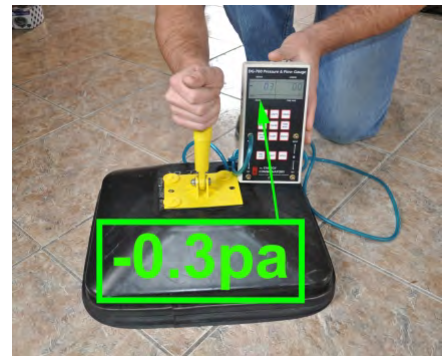
Perform pressure pan test after work is completed and compare to 'before' reading
