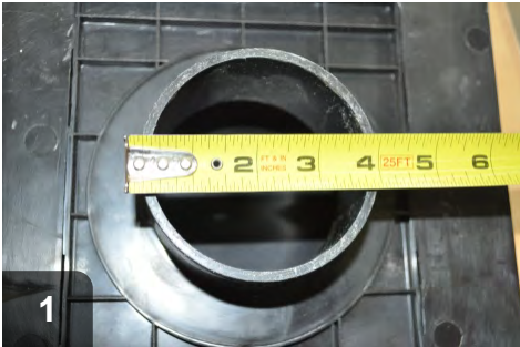
Measure the termination fitting to determine proper hole diameter (in this case, 4")
