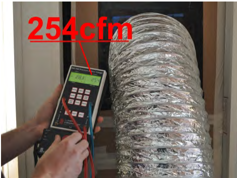
Run duct blaster test before beginning work and record result
