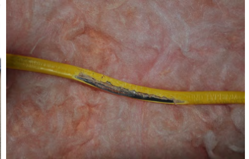
Inspect work space for hazards and safety concerns before work begins
