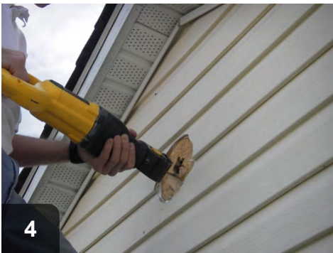
Since opening is larger than most hole saws, precision cutting is important
