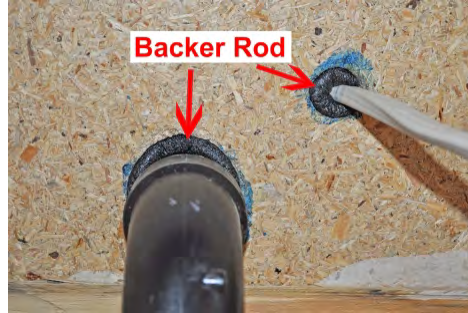
Infill with backer rod
