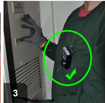
3 All workers should wear personal ambient CO monitors and halt work if levels exceed 35ppm
