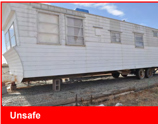
Unsafe Unstable mobile homes are unsafe work environments. Do not crawl under mobiles that are not stabilized
