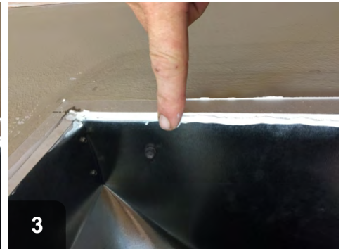
Wipe the caulk into the joint and smooth it as you go
