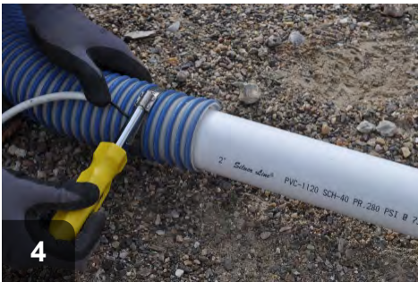
Attach grounding wire to fill tube
