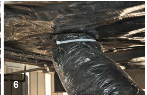
6 Secure insulation and casing in place using tie band and band tensioner
