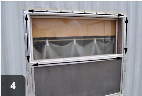
4 Run sealant bead around entire sash to seal glass from the interior
