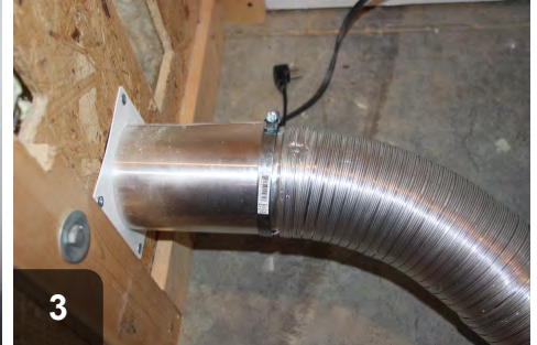
3 Attach approved vent material to termination vent. Termination vent may need to be trimmed.
