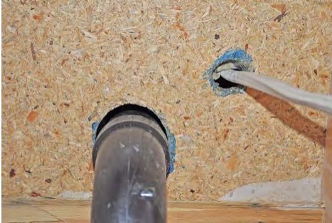
Prepare work space by removing any insulation
