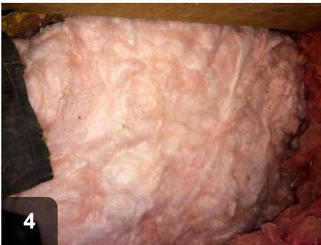
Replace or reinstall fiberglass belly insulation
