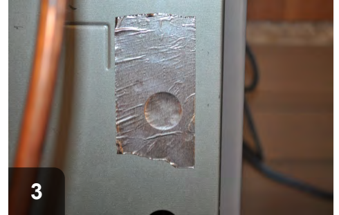
3 Fully cover holes with tape to seal completely
