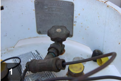
1 Propane - Ensure gas valve is open at the tank and there is fuel in the tank.
