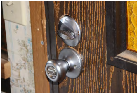
Doors should open easily from the inside, with no key or special knowledge of the locking system.
