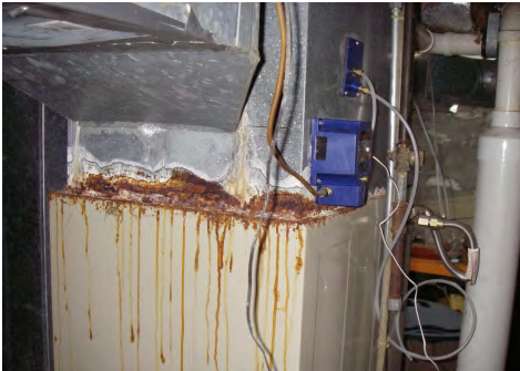
Assess existing combustion appliances for damage and replace when necessary
