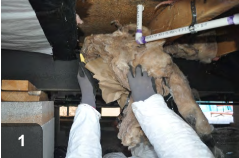
1 Remove old rodent barrier and insulation
