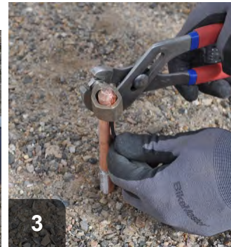
Attach grounding wire to rod with coupler
