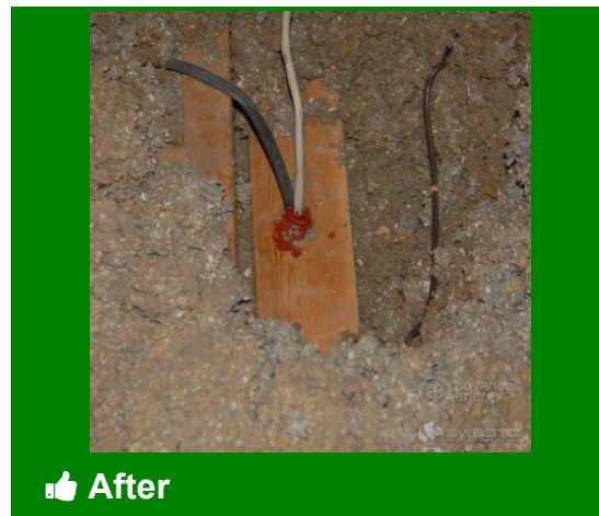
Sealed wiring penetrations through top plate
