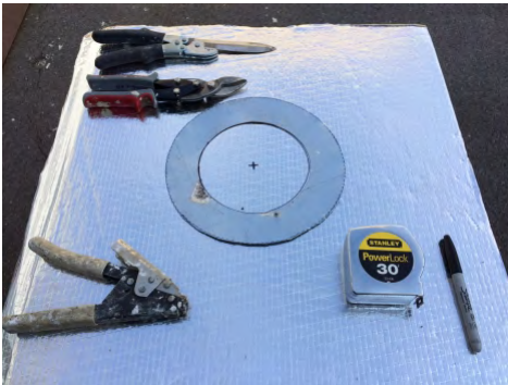
Select a backer ring and flex duct installation tools
