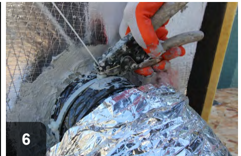
6 Secure with properly tensioned zip tie.
