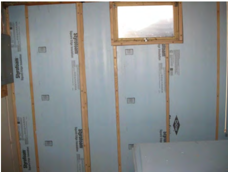
XPS insulation board is a non-absorbent insulation option
