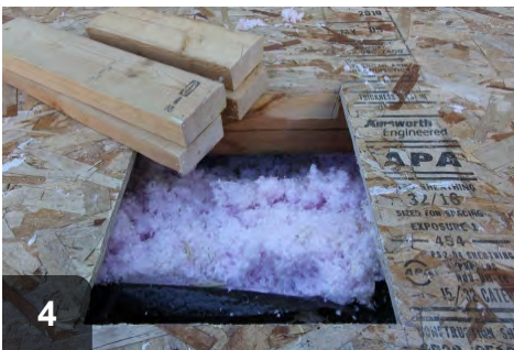
4 Cut four 2X4 blocks to support the patch
