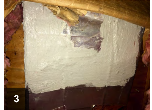
Overlap foil tape with mastic by at least one inch on all sides
