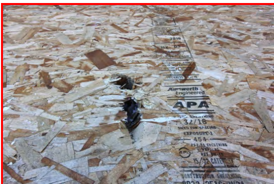
Remove floor coverings from damaged area
