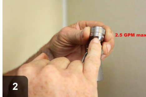
2 Replace with 2.5 gpm maximum shower heads
