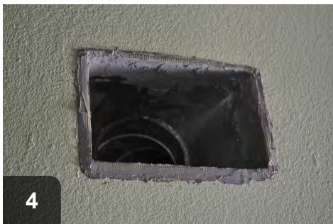
4 Apply mastic over mesh tape to create heat resistant, durable bond
