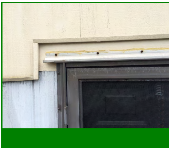
Install and caulk drip caps over manufactured home doors
