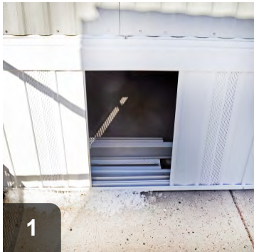
If skirting overlaps siding, remove skirting
