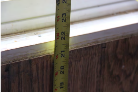
Window sill height should be no more than 44 inches from the floor.
