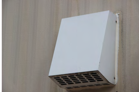
Through the wall exhaust fan sealing.
