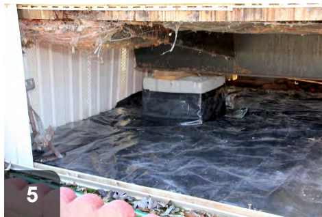
5 Remove tools and excess material
