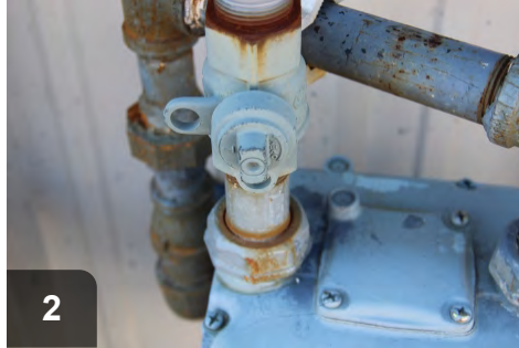
2 Natural Gas - Ensure the valve on the meter is on.
