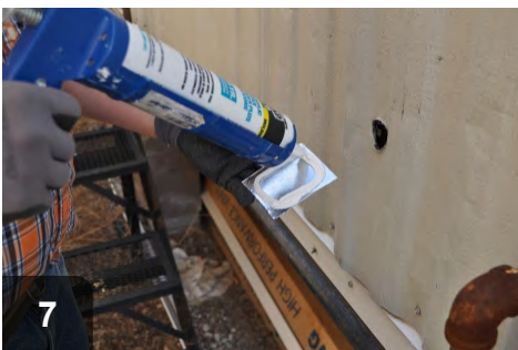
Apply sealant to back of patch to maintain air barrier
