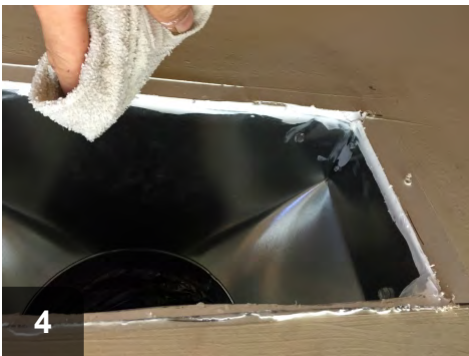
Wipe away excess caulk (use water on siliconized acrylic, alcohol on silicone, and solvent on polyurethane caulk)
