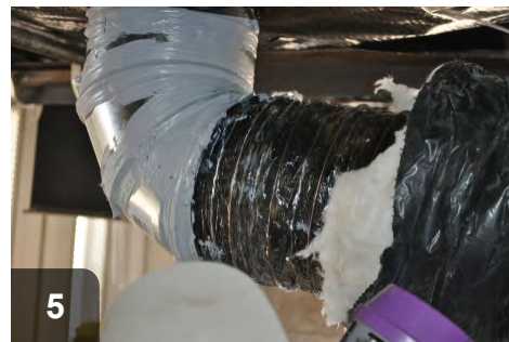
5 Slide inner liner onto flange with sealant
