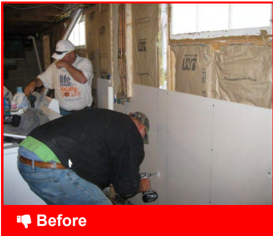
Kraft-faced fiberglass insulation is absorbent
