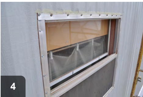
4 Sash should be completely clear of debris before moving forward with installation
