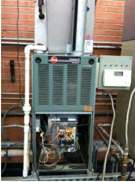
Cat I 80% efficiency furnace
