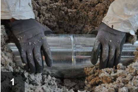
1 Realign and join ducts to create a smooth transition
