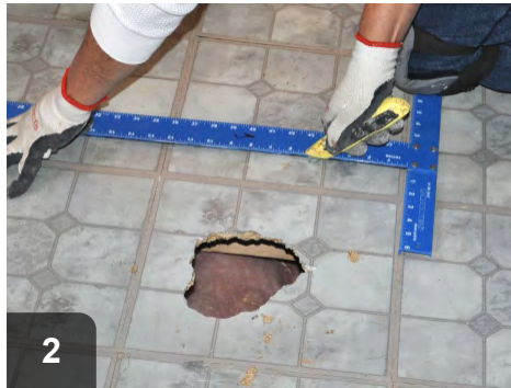
2 Mark damaged area to be removed to create most efficient patch
