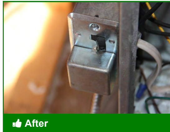
Appliance is set to ON at the disconnect, and can now fire.
