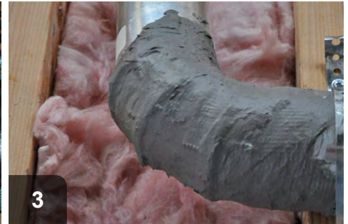
3 Apply UL 181 mastic to seal joint
