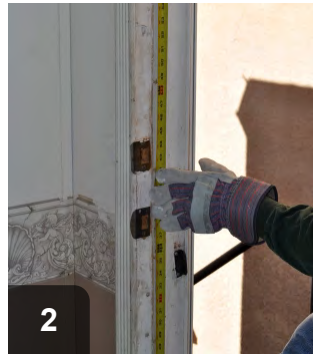
2 Measure door jamb for weatherstripping
