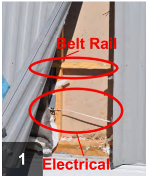
Obstacles should be noted and planned for--insulation should be tucked behind belt rails
