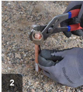
Attach grounding wire to grounding rod with acorn coupler
