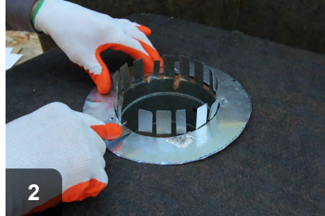
2 Place backer ring inside duct board. Insert collar and bend tabs into place.
