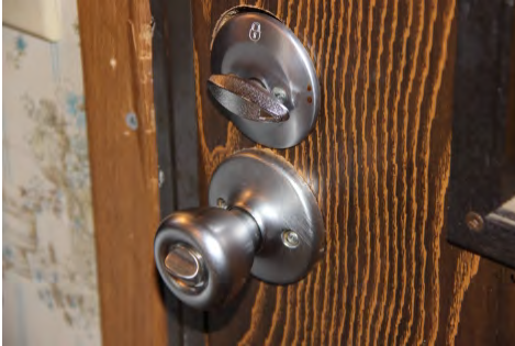
Door has a lockset that is easily operable from the inside without a key or special instruction.
