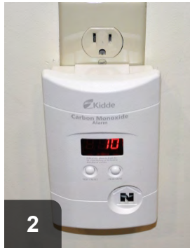
2 All homes should have CO monitors installed. If levels are elevated, look for the source
