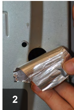
2 Removable foil tape should be used to seal
