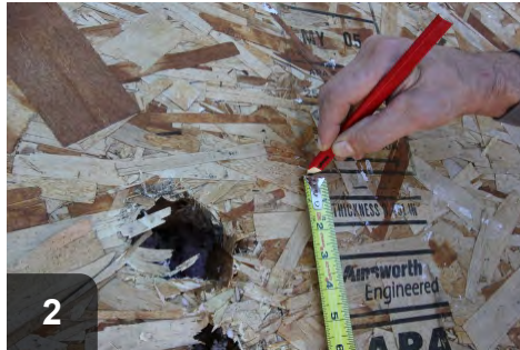
2 Mark the joist locations on either side of the damaged area
