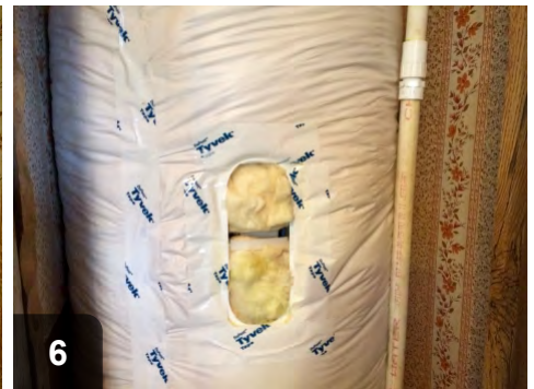
6 Cut out around drain valve, P&T relief valve, and thermostats. Do not cover combustion access or air supply on gas units
