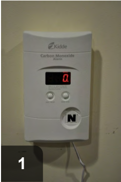
Mount alarm to wall close to bedrooms
