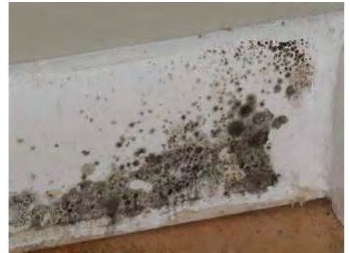
Unvented space heaters can create moisture issues in homes, leading to black mold
