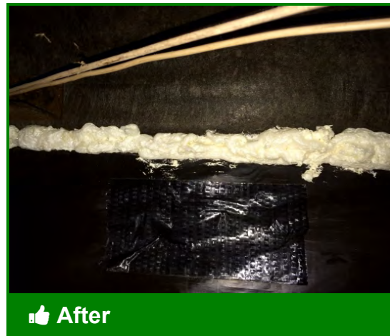
Completed air sealing at marriage line
