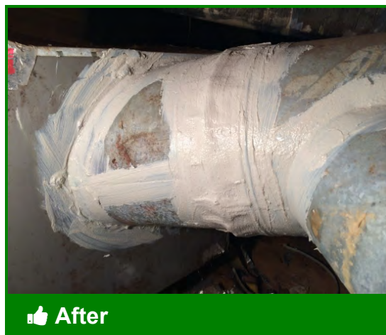
Mastic and mesh tape used to seal metal ductwork
