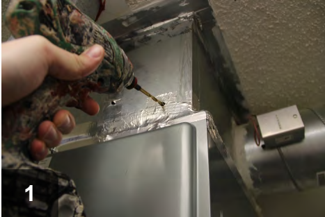
Drill holes being careful not to damage the evaporator coil.
