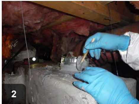
2 Apply mastic to metal collar
