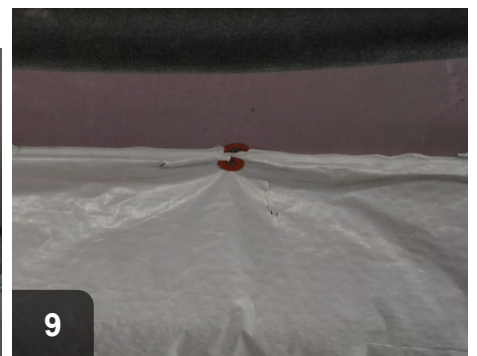
9 Insulation around ducting should be securely fastened and sealed to maintain air barrier
