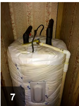
7 Use remaining insulation for the top of electric water heaters. Tape up seams in the vapor barrier. Insulate water lines
