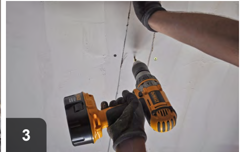
Cut drywall and fasten in place
