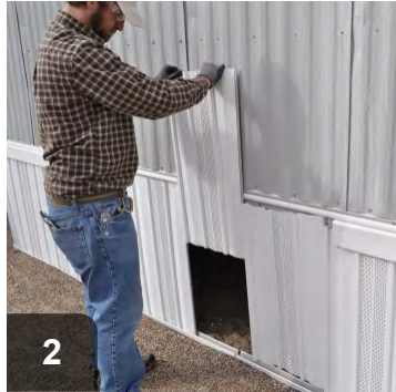
Reinstall skirting, if necessary
