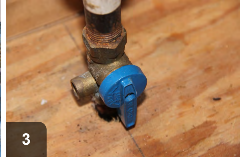
3 Ensure gas valve is open at the appliance.
