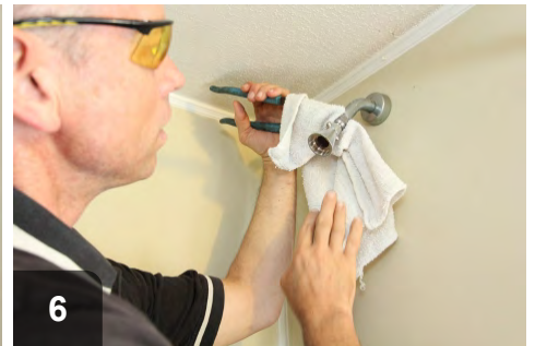
6 Tighten the shower head using an adjustable wrench or tongue-and-groove pliers and a rag to protect the finish.
