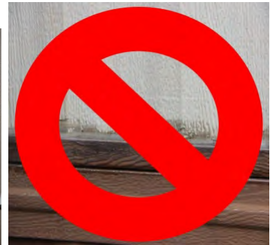
Do not seal intentionally ventilated wall assemblies!
