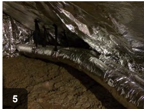
5 Wrap duct with R-8 insulation. Seal seams in insulation vapor barrier with UL-181 listed foil or Mylar tape
