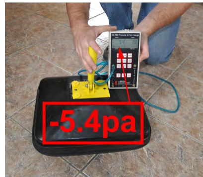
Perform pressure pan test on ductwork before beginning work. Record result
