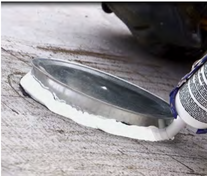
Insert 6" plug and seal around the perimeter of the opening.
