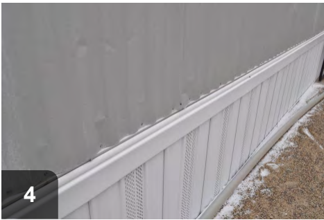
Verify that siding and skirting have not been damaged and show no signs of bulging
