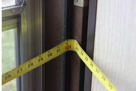
Egress doors are the proper width for egress.
