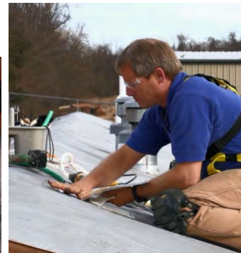
Apply a 14"x14" self adhering roof patch on top of the sheet metal patch.
