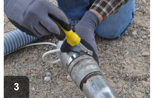
Attach grounding wire to metal fill tube with metal coupler
