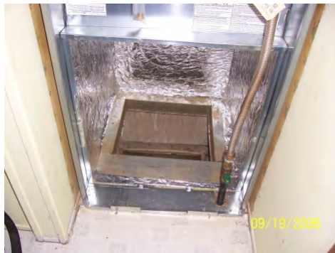
Remove the furnace panel. If the plenum to trunk connection is accessible here, complete sealing from this point
