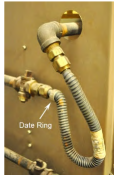
Inspect flex lines for damage, and check date on ring for pre-1973 hardware
