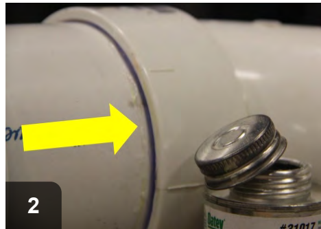
PVC-to-PVC connections should use PVC primer and cement.
