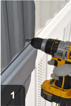
Using new fasteners, reattach paneling
