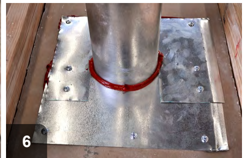
6 Fasten rigid material to cover penetration and seal against flue with caulk
