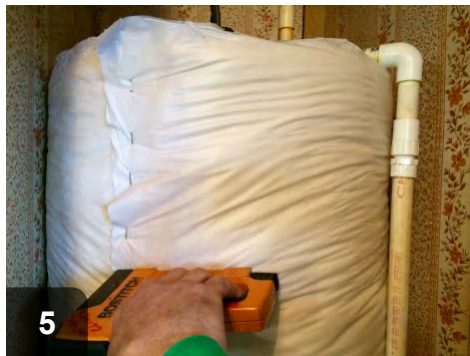
5 Staple the flap to the blanket with outward clinching staples or use long zip ties to secure the blanket in place
