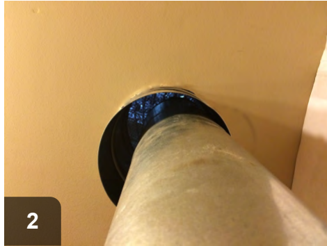
2 Cut hole in ceiling and mount high/low vents to framing
