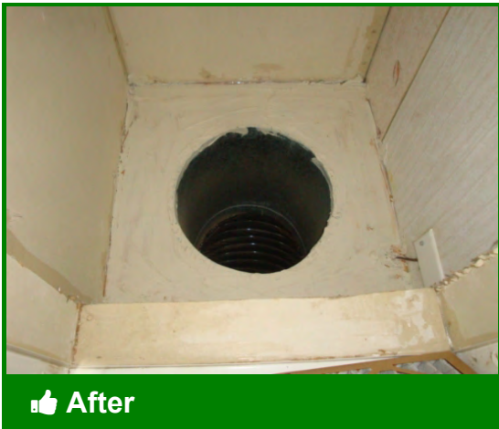
Closet prepared for furnace installation
