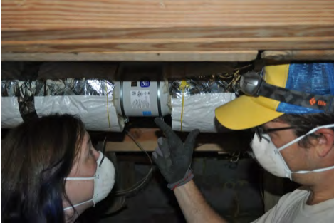
In homes with booster fans, occupant should know location and how to clean
