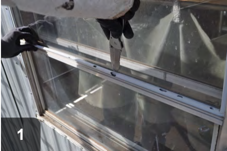
1 Remove exterior stops--these will probably not be salvagable
