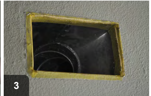
3 Cut mesh tape to fit around duct boot and cover gaps
