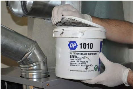
GOOD: Wear nitrile gloves when handling mastic
