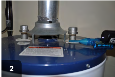
2 Complete spillage test using chemical smoke pencil or mirror
