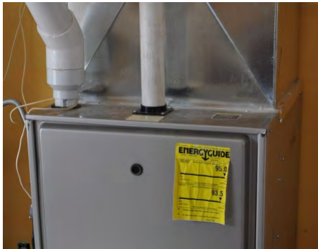
Two-pipe 90% efficiency furnaces are viable replacement appliances
