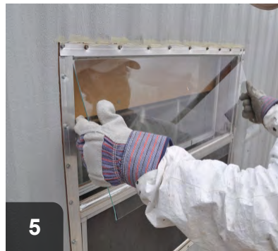
5 Install new glass, ensuring 1/8" gap from frame on all sides
