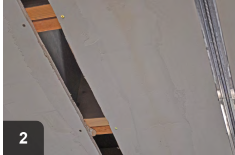
Prepare the hole by cutting the edges clean and square
