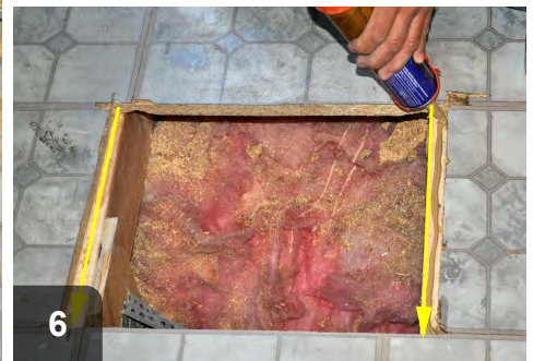
6 Apply sealant to mounting surfaces
