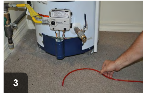
3 Place test hose by combustion appliance
