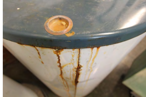
Inspect for rust, corrosion, and leaks
