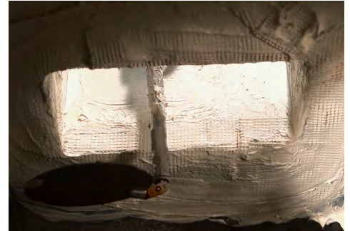
Seal the boot to the trunk line using mastic and mesh tape. An inspection mirror can make this easier.
