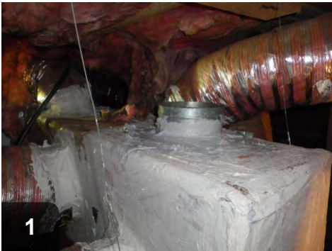
1 Fasten collar into plenum with screws that reach through the tabs and plenum into a backing ring. Apply mastic liberally
