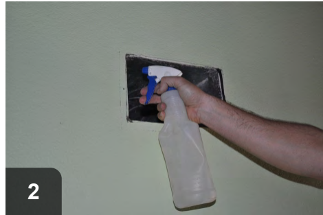
2 Wet the edges of the drywall to ensure a good bond
