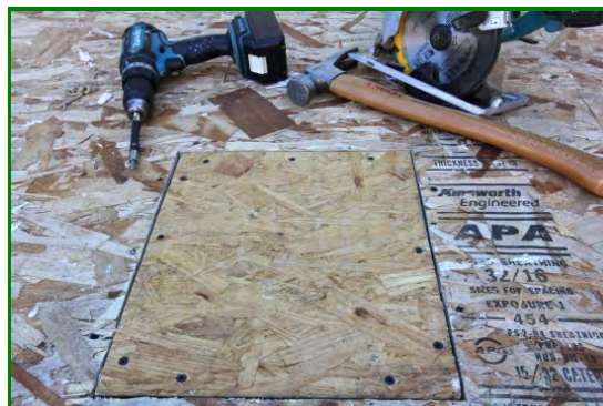
Completed floor repair
