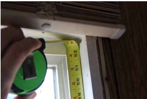
Windows are the proper height for egress.
