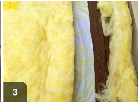
3 Cut the insulation off at the mark. Peel away the excess insulation, leaving a flap of vapor barrier
