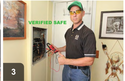
After electrician verifies wiring is safe, proceed with retrofit work
