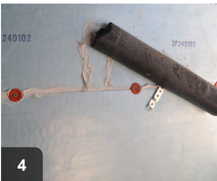
4 A rigid air barrier should be securely in place so prevent sagging, gaps and penetrations should be sealed
