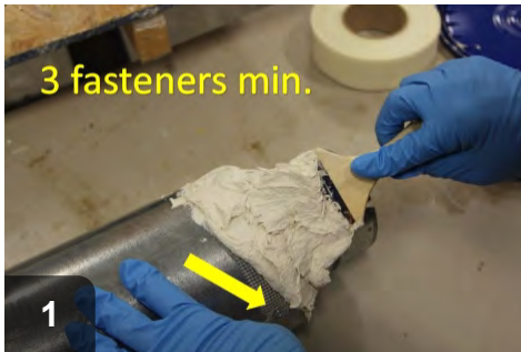
Round metal-to-metal connections require fiberglass mesh tape and 3 mechanical fasteners minimum.
