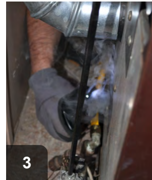
Test for spillage--should not exceed 2min. If 2min are exceeded, mitigate.
