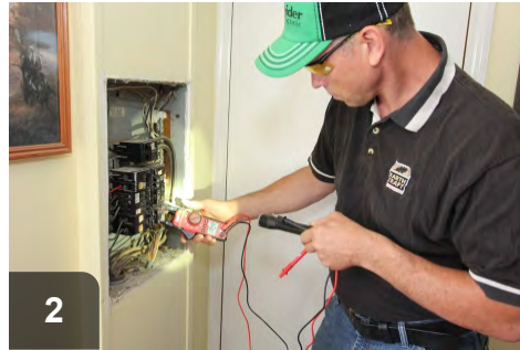
Have a certified electrician inspect every aluminum wire connection in the home
