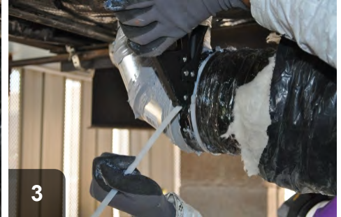
3 Using band tensioner, securely attach liner in place with tie band
