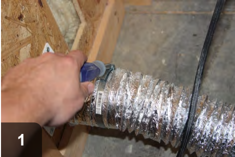
1 Disconnect existing vent pipe from termination. If hose clamp is installed, save for reuse.
