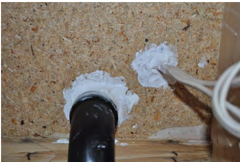
Visually inspect to verify no gaps remain
