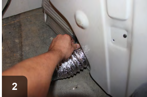
2 Disconnect existing vent pipe from dryer.
