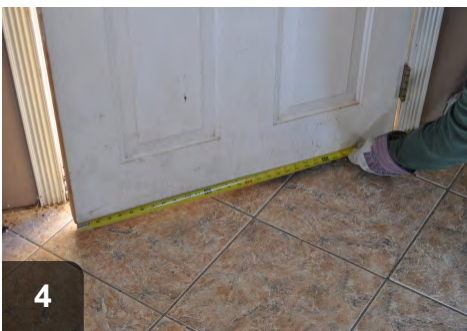
4 Measure bottom of door for door sweep
