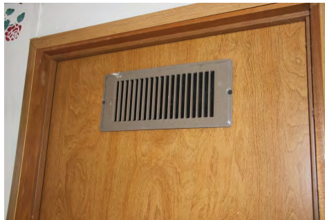
If pressure relief is needed, it can be provided by a through the door transfer grille.
