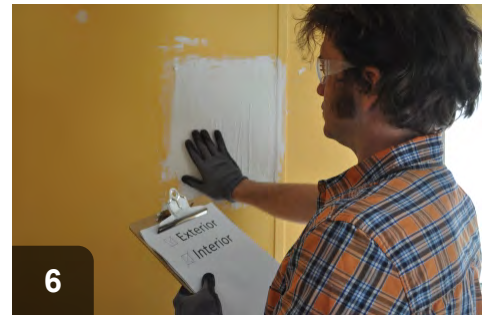
6 Verify that patches to both interior and exterior have been completed before beginning installation
