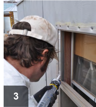
3 Apply sealant to sash with bead at least 3/16" wide
