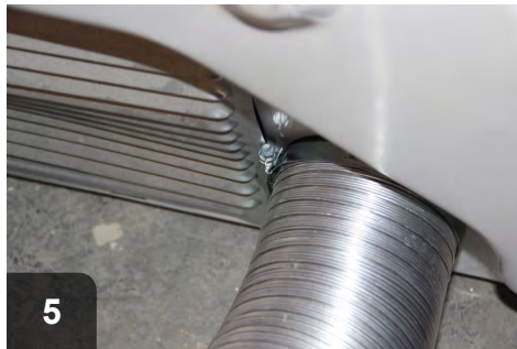
5 Connect vent pipe to dryer.
