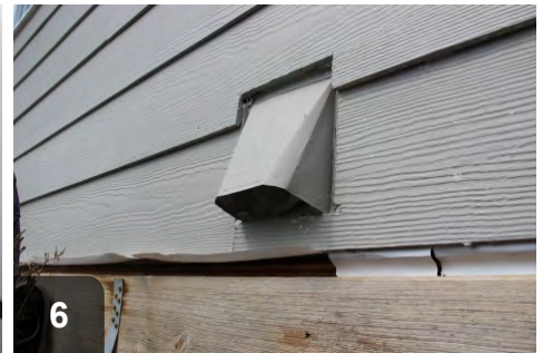
6 Dryer vents to outdoors, and exhaust damper is functional.
