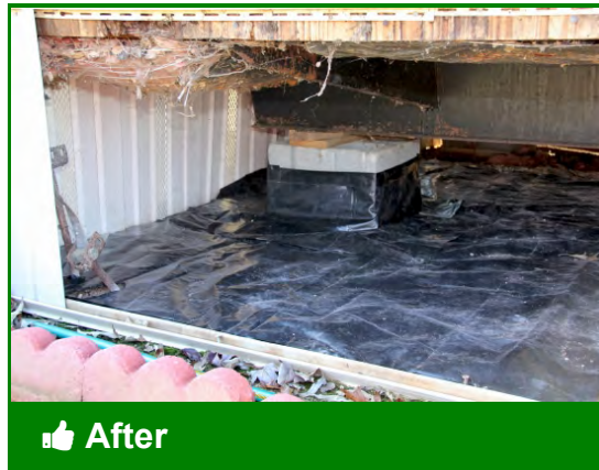
Manufactured home crawlspace with complete ground vapor barrier
