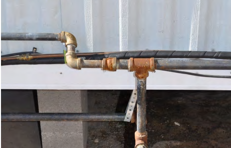
Inspect exterior gas and oil lines for leaks and damage
