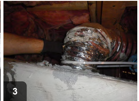
3 Install duct liner onto collar and secure with properly tensioned zip tie
