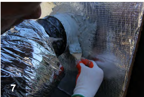
7 Coat seam with mastic
