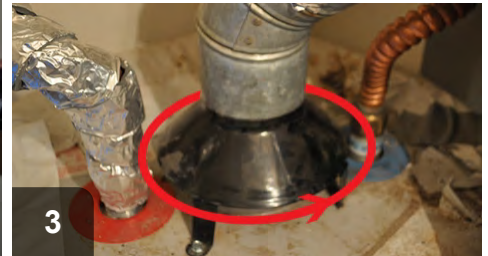
3 Test for spillage on all sides of draft diverter. Check spillage on all atmospheric combustion appliances
